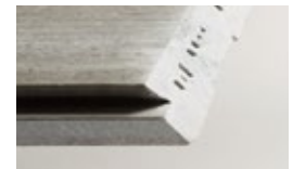
Installation order (2) Cut the edge of the panel at angle of 45 degrees. (Use a circular saw that can cut a panel at angle of 45 degrees)
