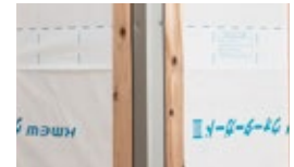
Installation order (1) Install slim metal corner
